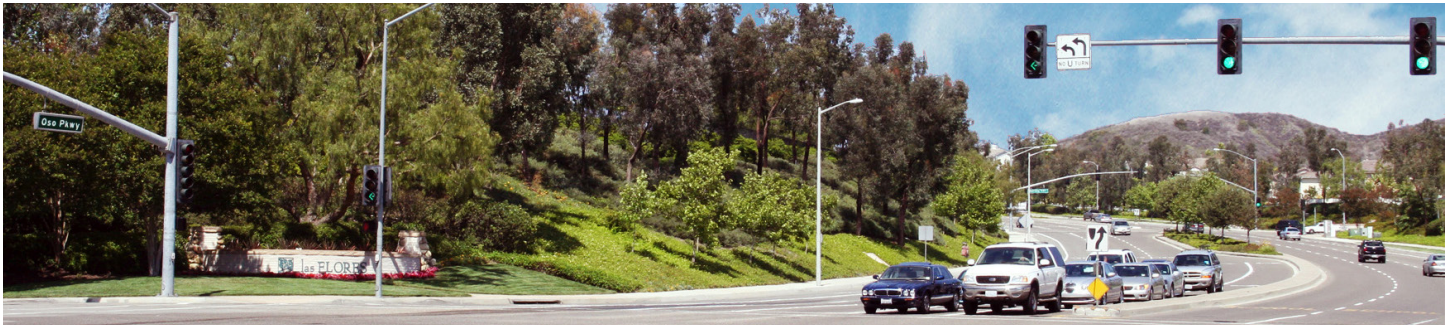
Signal synchronization on Oso Parkway keeps traffic flowing.
