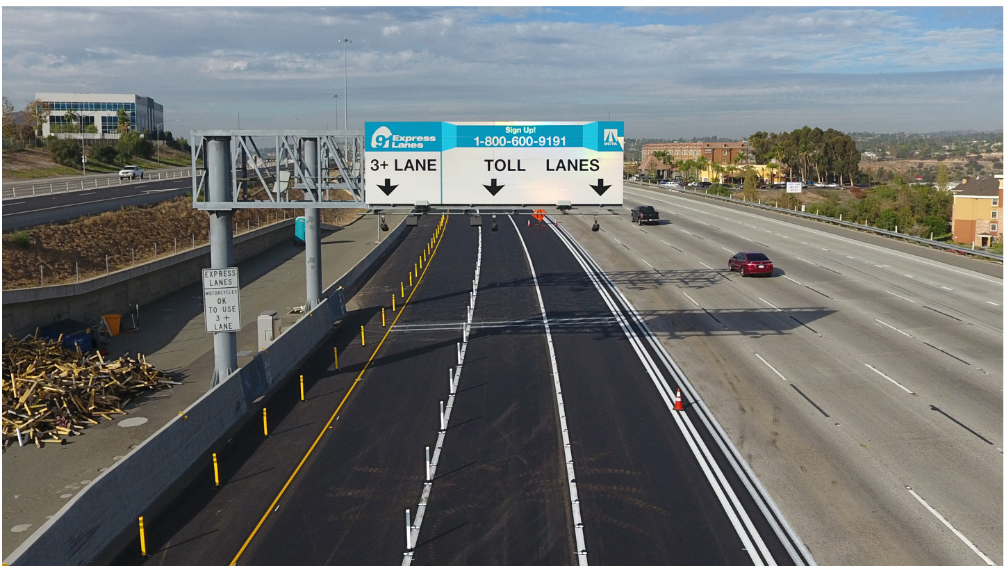
The Pavement Replacement Project on the 91 Express Lanes was completed in 2016.
